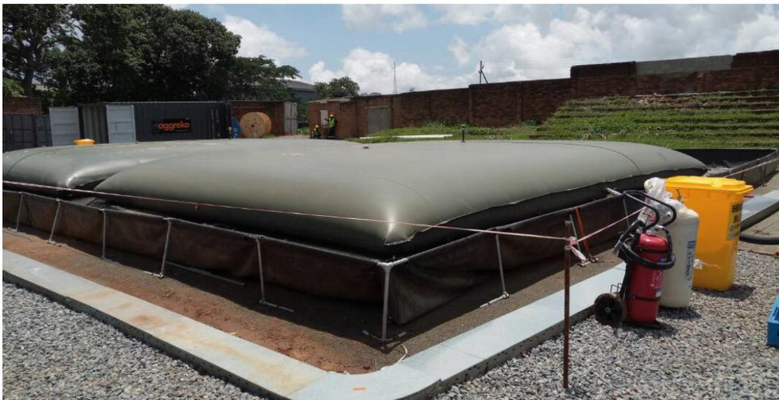
*Above: 2 x 100m<sup>3</sup> Bladder / Berm system installed Malawi, 2018; Image courtesy Aggreko Rental Power Services*
